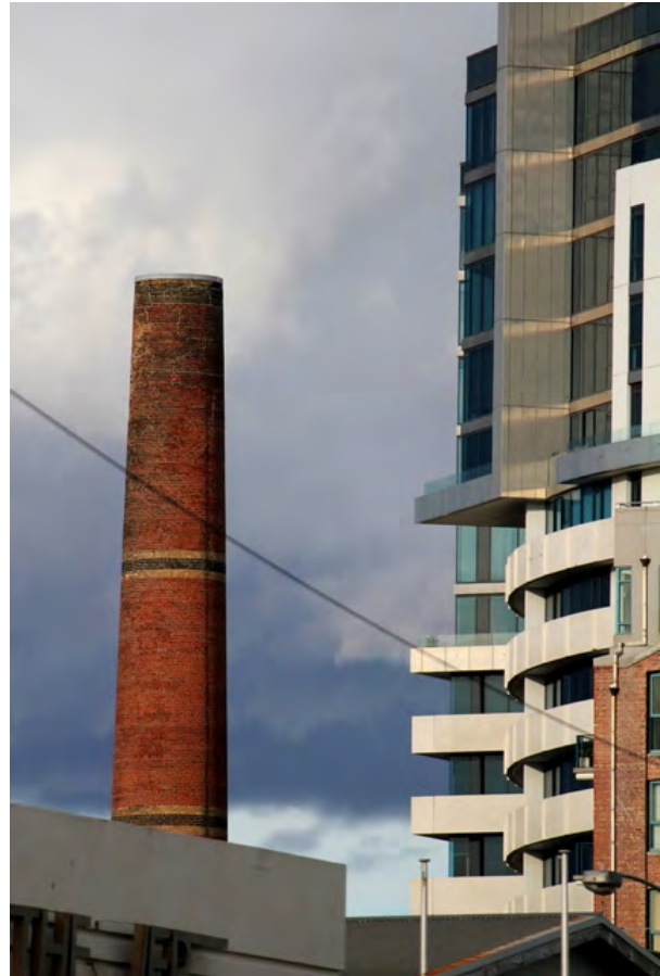
Former industrial sites and a former HMAS Lonsdale Navy Depot have been converted into apartments. Photograph by Kate Kelly.
